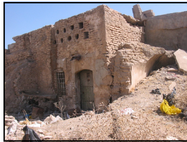
Dilapidated homes continue to be a common scene in the Nineveh Governorate. Photo taken in April 2005 of a currently inhabited home by a large family in the district of Hamdaniya, Nineveh, Iraq.
